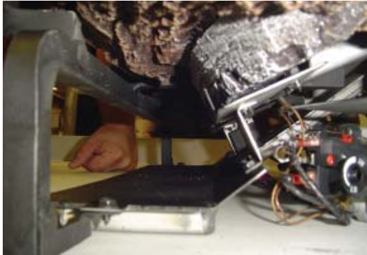
Figure 22C - Installing Right Front Log, Side View
